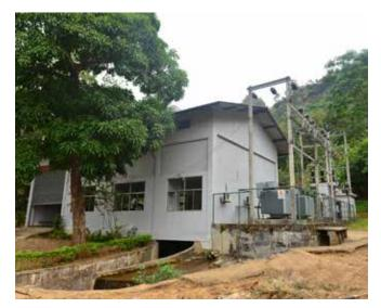
Installed capacity: 2.4 Mega WattsPenstock length: 950 MetersChannel length: 1,800 MetersNet head: 280 MetersElectro mechanical equipment Supplier: Global Hydro Electric, AustriaYear of commissioning: 2008Total production (FY 2014/15): 7,467524 kWhCatchment area: Kurunduoya and High Forest
