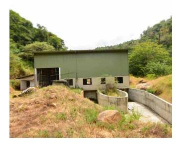
Installed capacity: 3.5 Mega WattsPenstock length: 470 MetersChannel length: 2,675 MetersNet head: 140 MetersElectro mechanical equipment Supplier:Global Hydro Electric, AustriaCatchment area:Piduruthalagala
