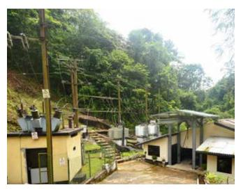
Installed capacity: **3 Mega Watts** Channel length: **880 Meters** Electro mechanical equipment Supplier: **Tianjin and Stamford** Year of commissioning: **2004** Total production (FY 2014/15): **11,716,713 kWh** Catchment area: **Hapugasthenna**
