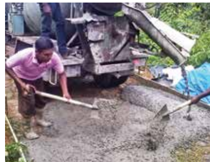
Construction of access road in progress
