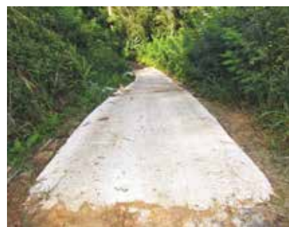
Part of the access road built at Raththurugala
