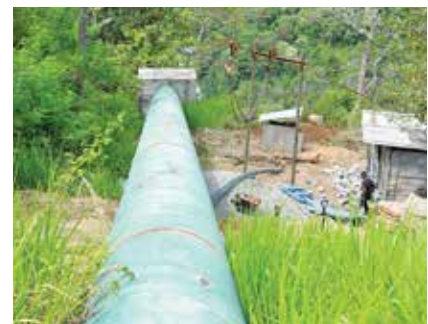
Padiyapelella construction in progress
